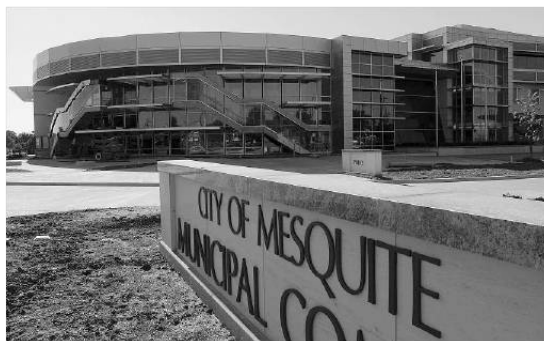
Mesquite's new city hall opens Monday with environmentally friendly interiors and an open plaza with terraced landscaping.
